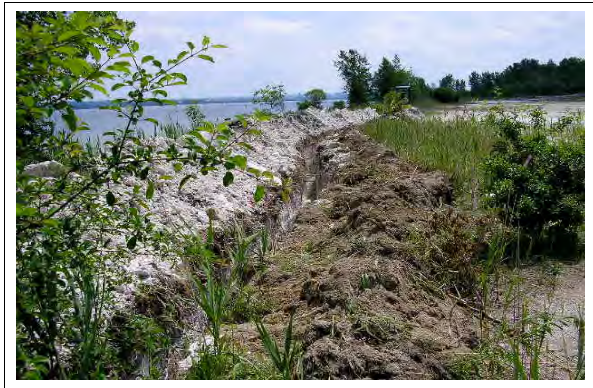
Photo 12 – Lengthwise view of TP-08. Date photo taken: 6/16/04
